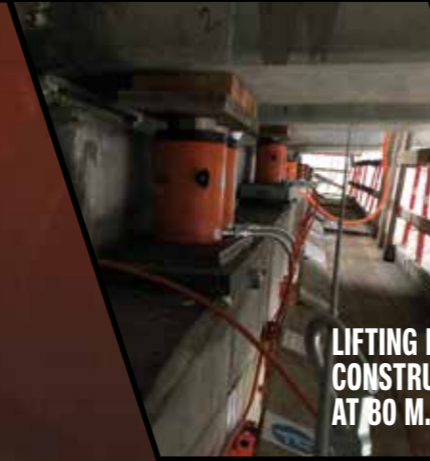
SUPPORTING A CONVEYER PLATFORM
